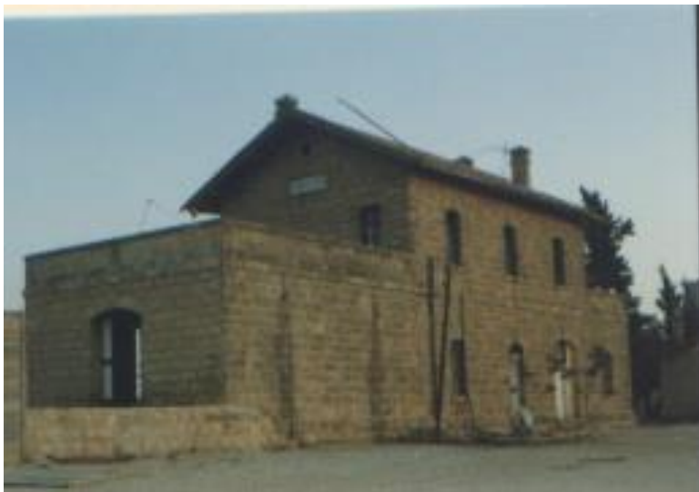
Figure 3: Jizeh Ottoman Station (Railway) General view (Waheeb, 2012)
